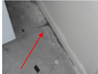
Along wall behind washer
