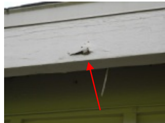
South exterior fascia
