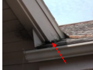
West corner of entryway roof
