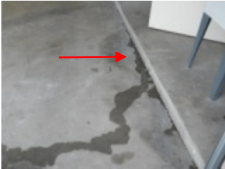
From below step-up in garage
