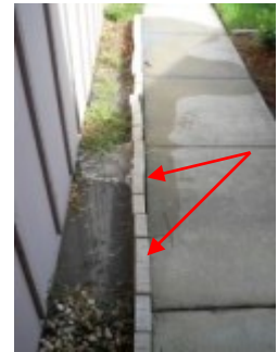
Along the East exterior wall
