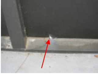
Base of west panel wall
