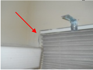
Corner bead of west living room window
