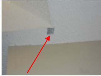
Corner bead along skylight
